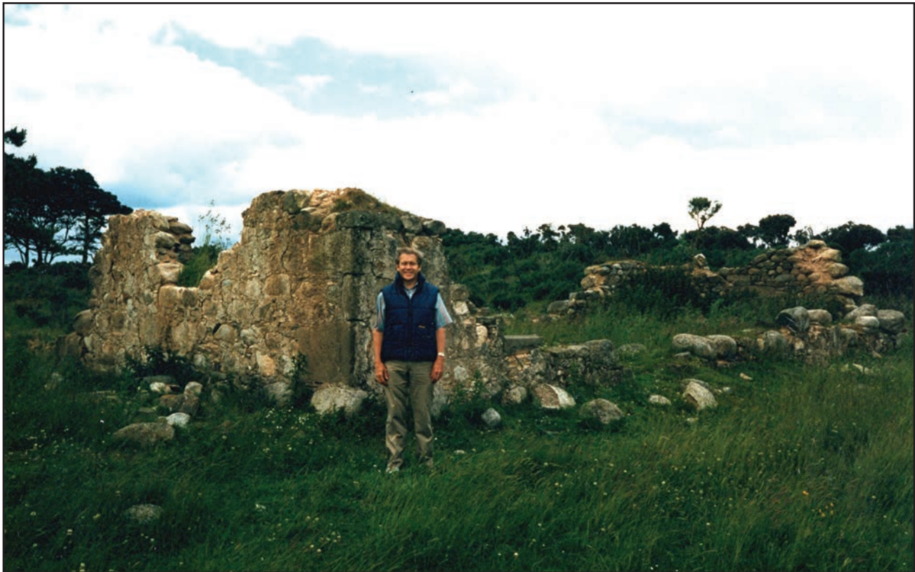
Only two walls and a few piles of stones remain of this old crofters' cottage in Balnahaugh. It was owned by a MacKenzie family, which might have been David and Isobella MacKenzie
