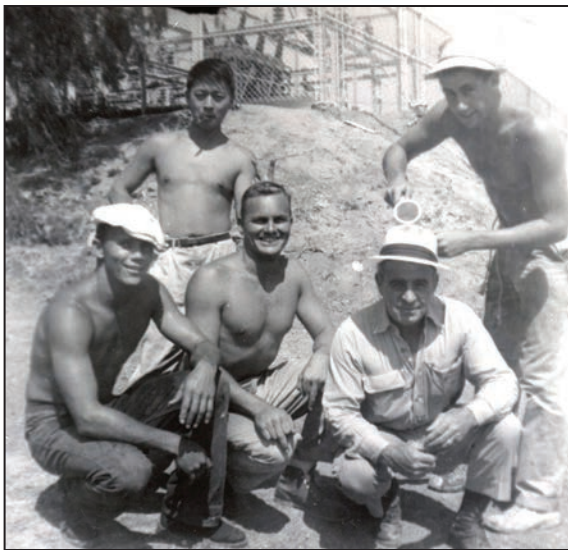
Summer Work Crew San Diego Gas & Electric Company
